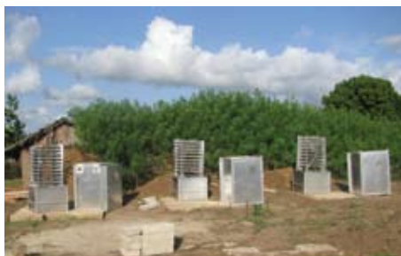
Loose-standing parts of the solar ice cooling system before assembly and installation
