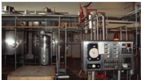
A milk processing plant at Kitale
